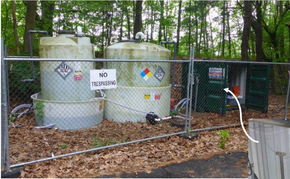
Figure 7. Example phosphorus inactivation dosing stations
